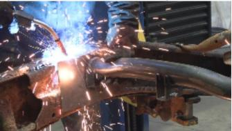
With the remaining two backing plates, push them onto the crossmember ends on the outside of the frame rails, and tac weld them into place.
