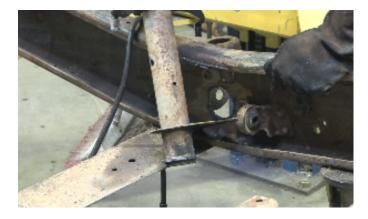
Grind the work area free of rust and debris, revealing bare metal, followed by coating the work area with a weld through primer to help prevent against further rust development.
